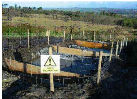
COMPLETED SETTLEMENT POND SYSTEM
